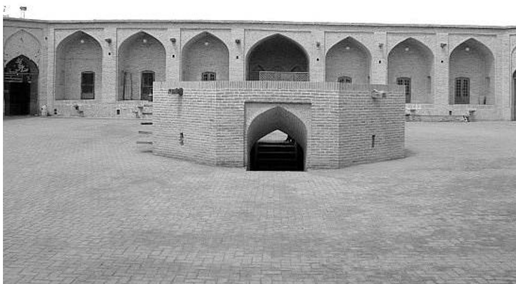
View of a renovated caravanserai
